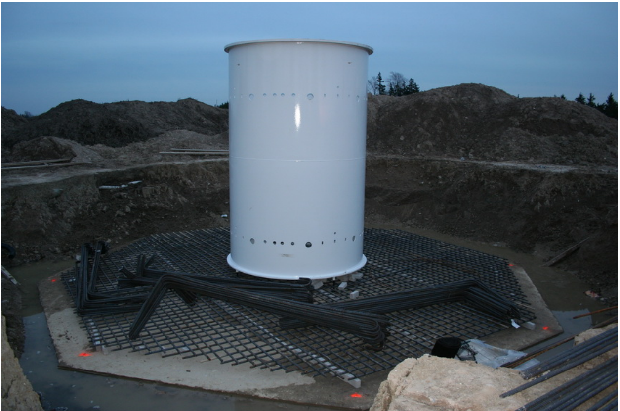
Foundation and anchor for a 50 meter tower.
