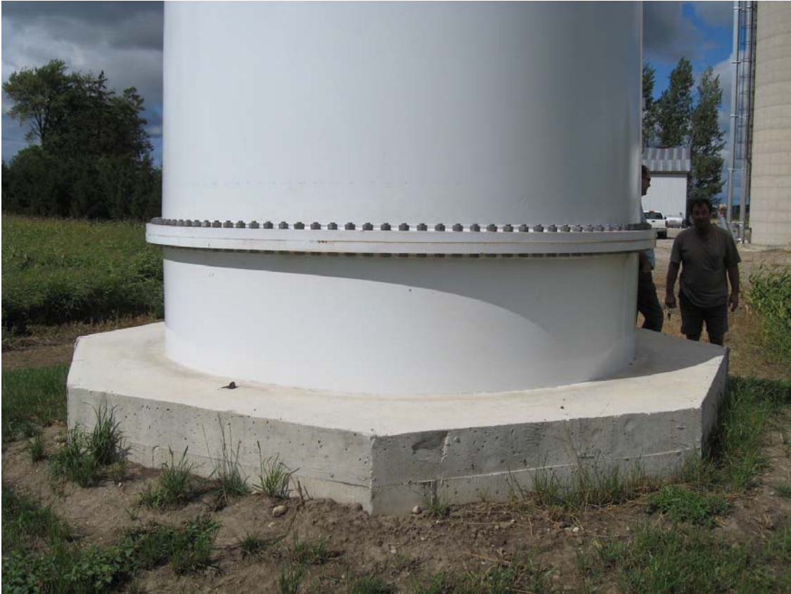
Foundation and tower foot of a 50 meter tower.
